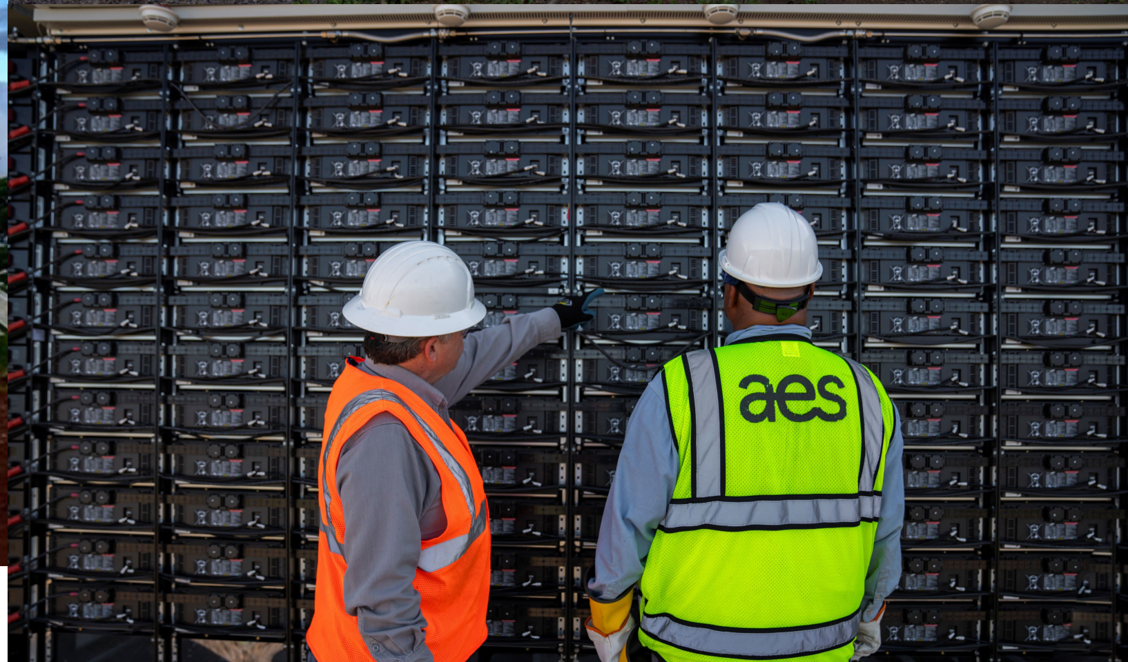
Battery Energy Storage System
